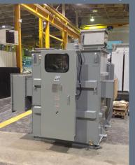
Left: Small power transformer with neutral grounding resistor
